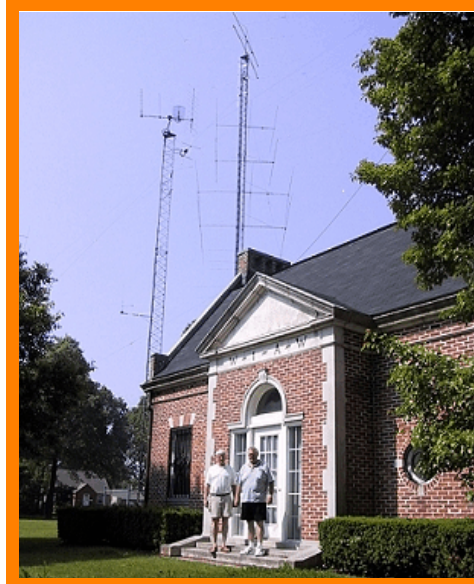
Gary KC2UBA & Bob W8GC on the front steps of W1AW building with 2 towers and several beams in the background
